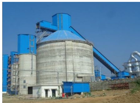
CLINKER SILO & UNBURNED SILO
