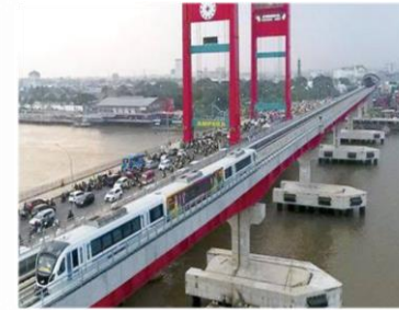
Light Rail Transit (LRT) Palembang
